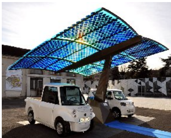
Photovoltaic SUDI shade is an autonomous and mobile station in France that replenishes energy for electric vehicles using solar energy.
